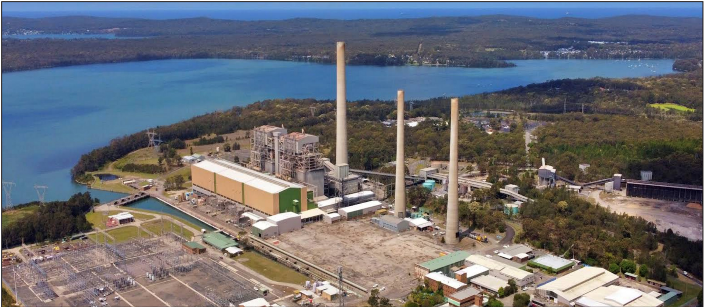
Vales Point Power Station. Source: Mountainscape Creative, 2021
